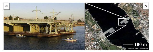
Fig. 7 – Side view from the north (photo a) and aerial view (photo b; ©Google Earth) of the Valide Sultan/Old Galata Bridge after 2000 with the two center sections removed.
